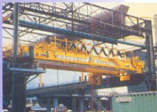
Motor control for travelling crane (Fos-sur-Mer).
